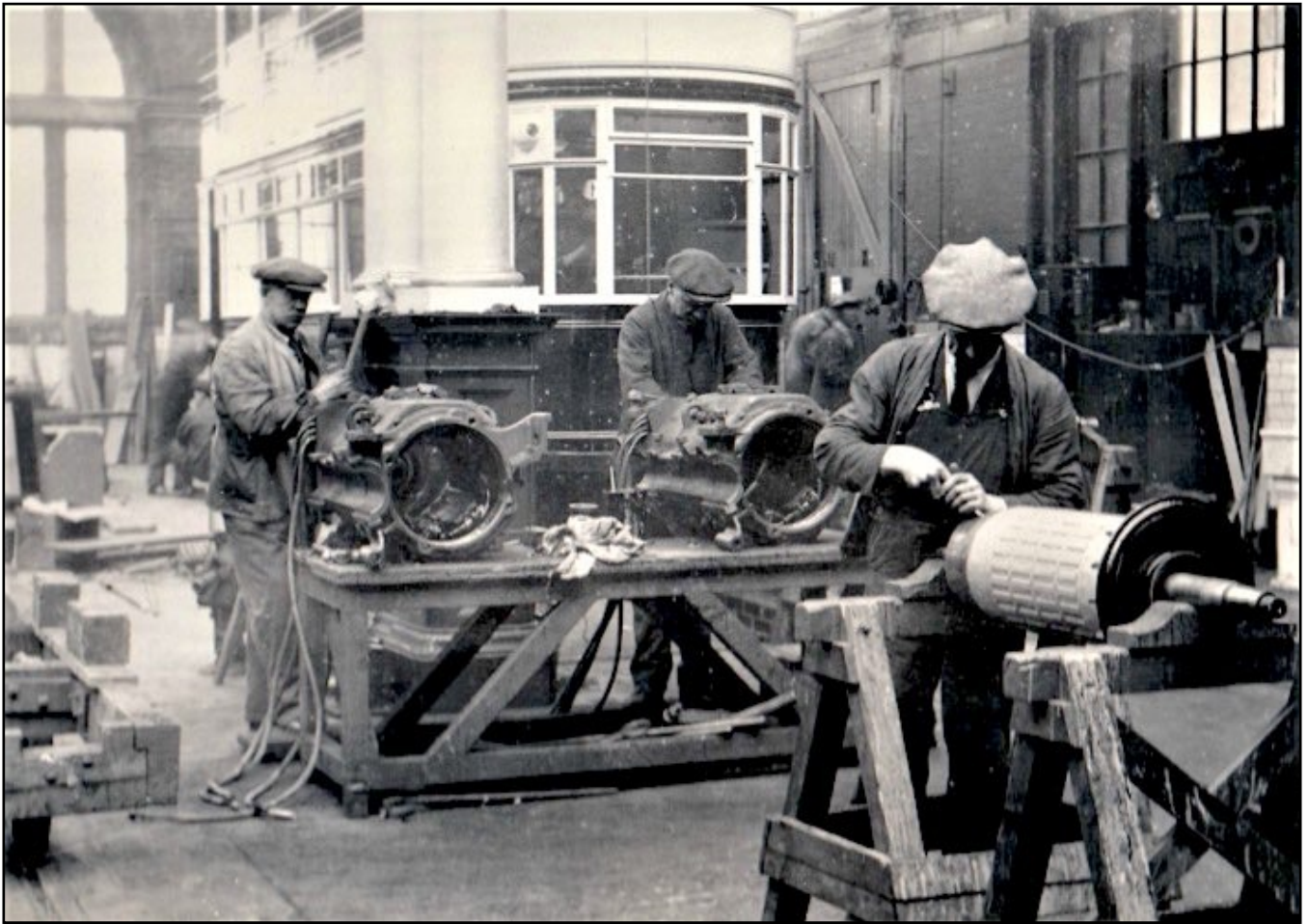
Motors being serviced showing armature in foreground
